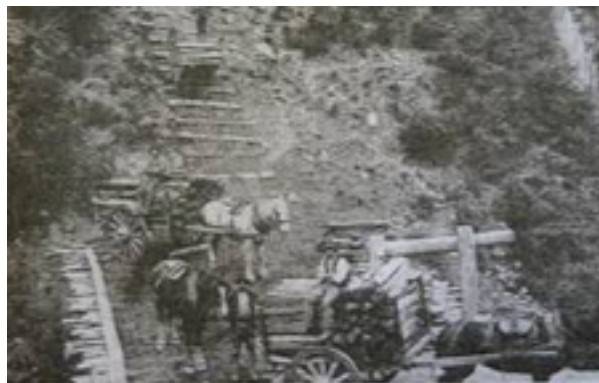
Timber cutting for the Township, and Mining at Walhalla.
